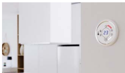
Controlli a parete Wall panel
